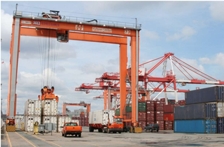
Figure 2: Rubber Tired Gantry (RTG)
